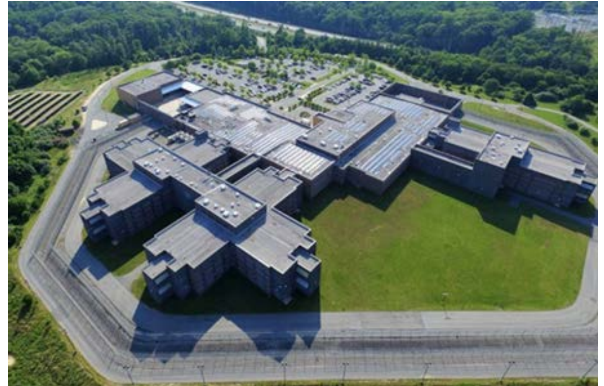
Montgomery County Maryland Correctional Facility Powered by a Campus Microgrid
